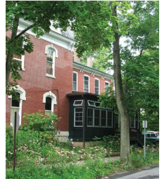
The addition to this historic home utilized the same proportion and orientation of window openings for a compatible design. The attention to details, ie the window trim, multiple panes and wood paneling, make the addition a success.
